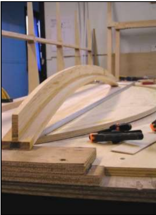
Two steam-formed members glued together, with a further laminated rib glued on.
