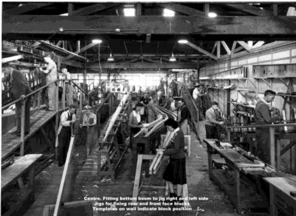
Centre. Fitting bottom boom to jig right and left side
